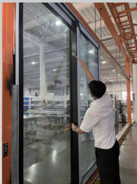
Install stationary panel side cover, use rubber hammer to hit it in if necessary
