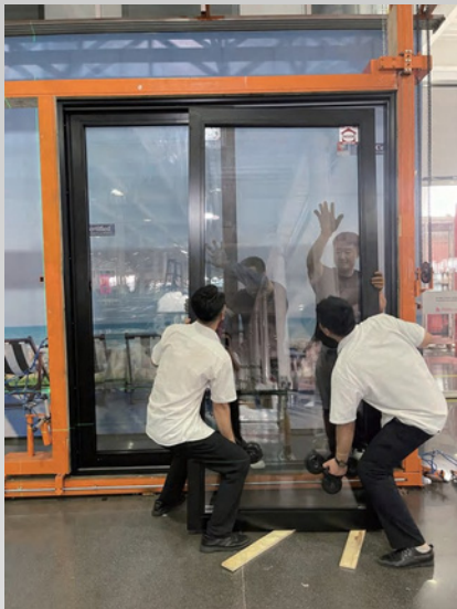
Insert the Sliding Door Panel into the top track
