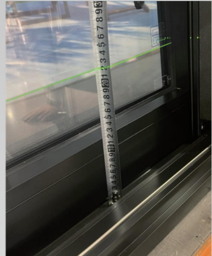
The laser line shows the horizontal level is same, no adjustments necessary
