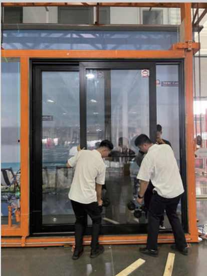
Lower the Sliding Door Panel onto the bottom track
