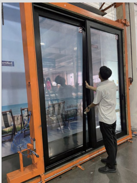
Install sliding panel side cover, use rubber hammer to hit it in if necessary
