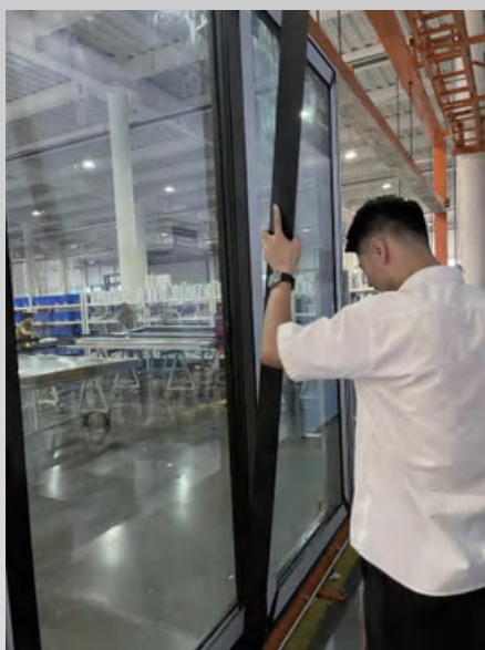
Install stationary panel side cover, use rubber hammer to hit it in if necessary
