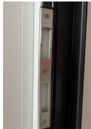
Loose the strike plate to move up or down
