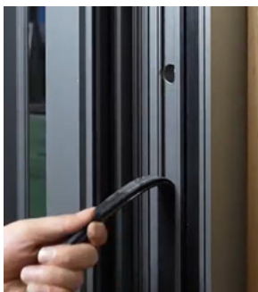
Remove rubber seal from the frame to show pre-drilled screw holes
