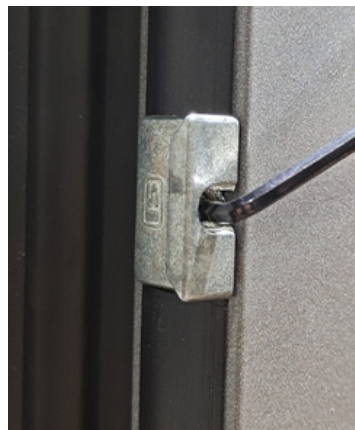
Loose the locking blocks to move up or down
