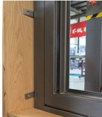
Screw the Metal Straps from the Interior
