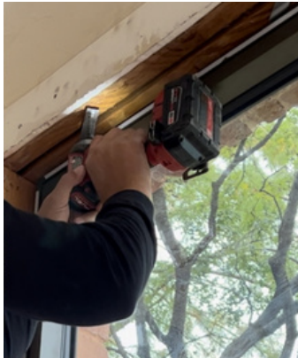
Screw the Metal Straps from the Interior
